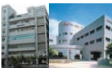
Taipei/Taichung, Taiwan Left: Taipei FA Center/ Right: Taichung FA Center
