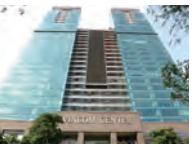
胡志明FA中心 Ho Chi Minh FA Center MITSUBISHI ELECTRIC VIETNAM COMPANY LIMITED
