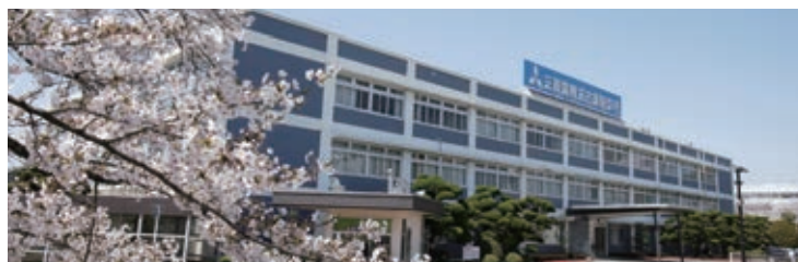
Mitsubishi Electric Nagoya Works
